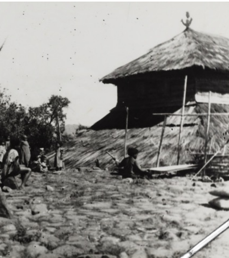
15) From the loom beneath onto the top of the roof. Weg richting de Keli Moetoe, Manggarai 1952. UBL: KITLV 164867 - http://hdl.handle.net/1887.1/item:834993
