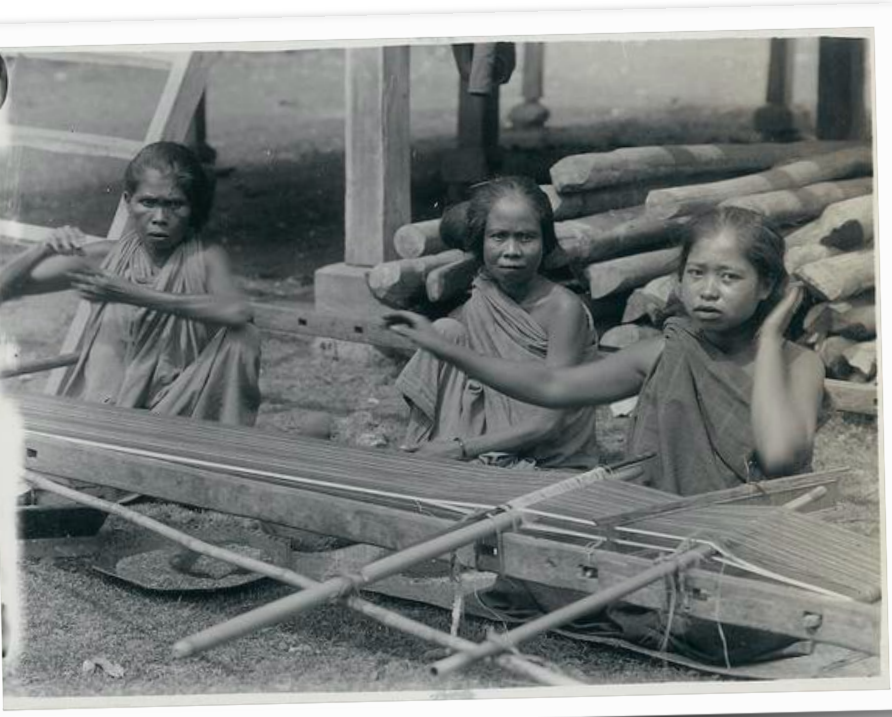
96) Horizontal warping device (alat melengkung) of the Bima on the western north coast on Flores in Kampong Pota, 1926. - Foto: UBL digital collection (KITLV 10985)
